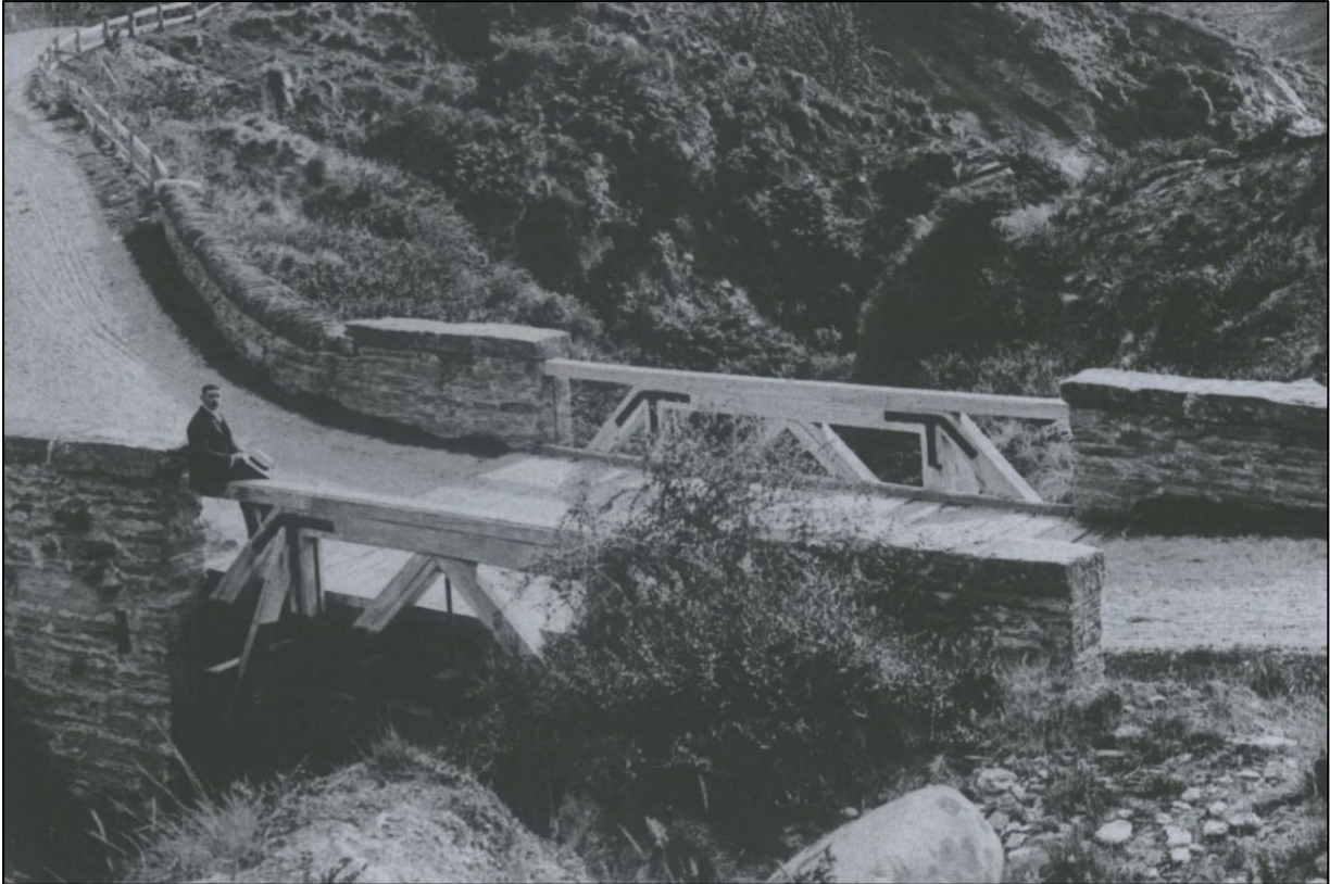
Figure 13. McChesney's Bridge circa 1903. 113
